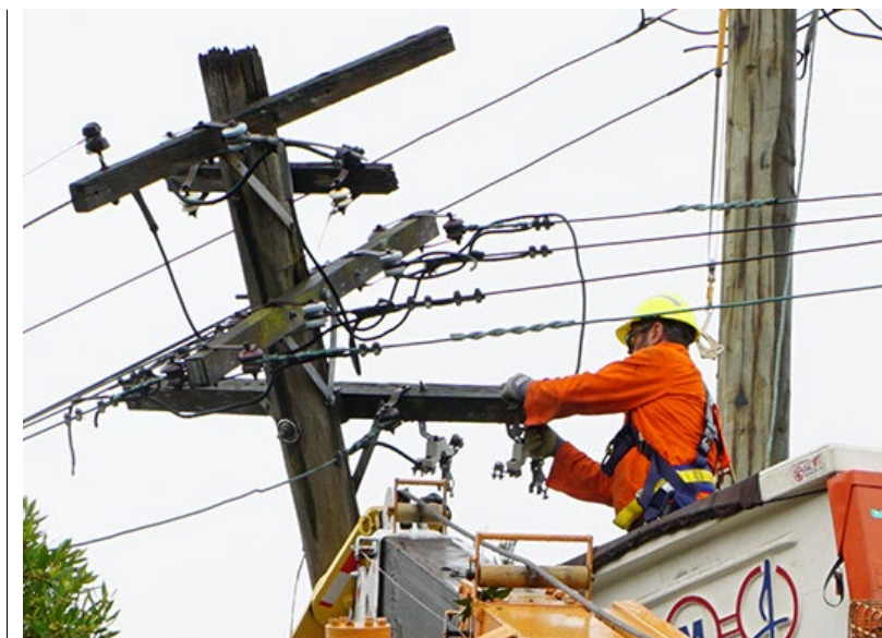
Ausgrid crew repair storm-damaged power pole.
