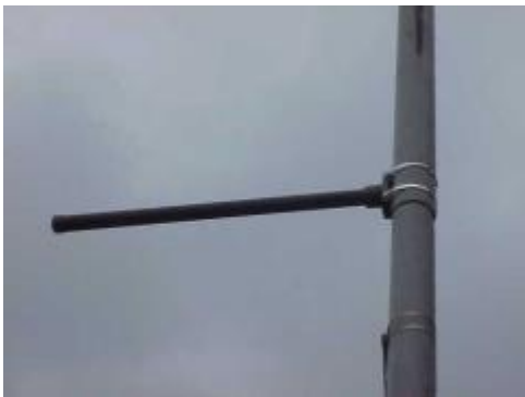
Figure 22: Banner support arm secured with approved stainless steel band clamps
