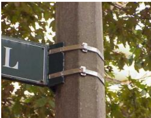
Figure 20: Road sign secured to a concrete column with stainless steel band clamps
