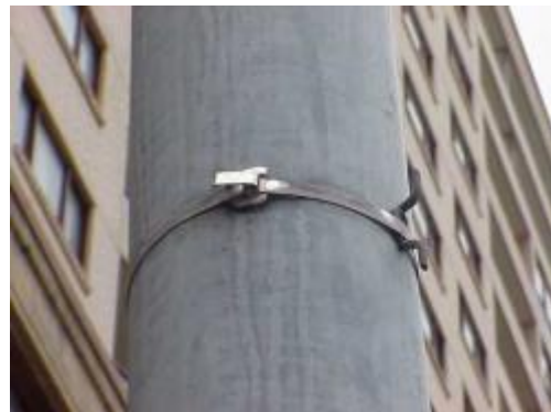
Figure 23: Banner base anchor secured with approved stainless steel band clamps
