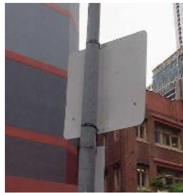
Figure 21: Sign inappropriately secured using plastic cable ties
