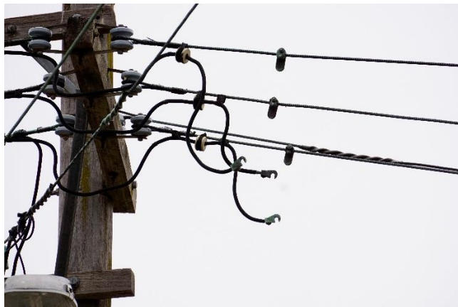
Figure E3: IDT links on LV mains
