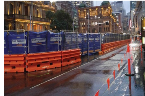
Portable noise screen used to mitigate noise
