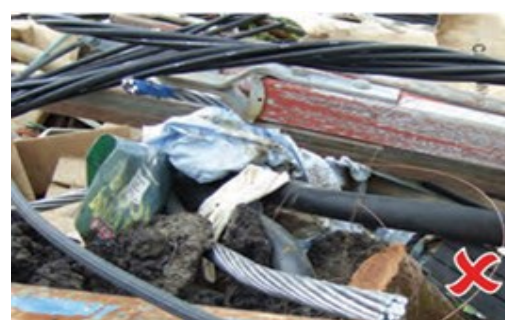
Segregate waste to avoid cross contamination Example of poor waste segregation
