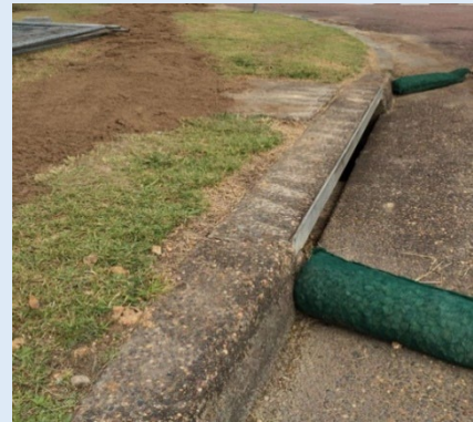
Grass filter strips can be used as an effective natural barrier
