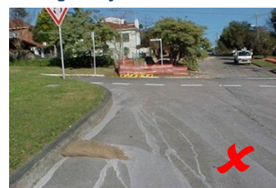
Saw-cutting slurry has not been contained effectively
