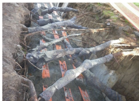
Where roots are exposed for extended periods of time (>24 hours), wrap larger roots (> 50mm diameter) in jute mesh or hessian and keep moist
