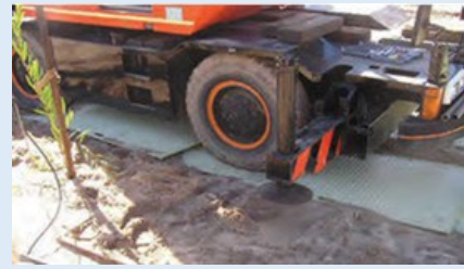
Temporary construction mats help minimise ground disturbance
