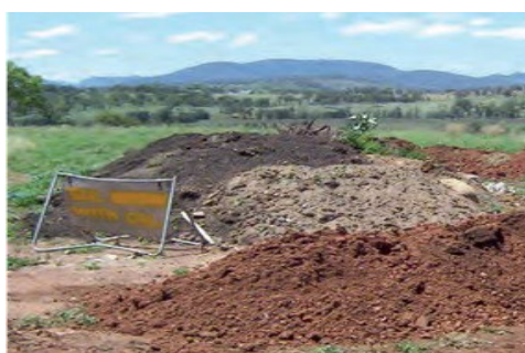
Segregate waste to avoid cross contamination Example of poor waste segregation
