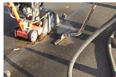
Wet-vac used to collect saw-cutting slurry
