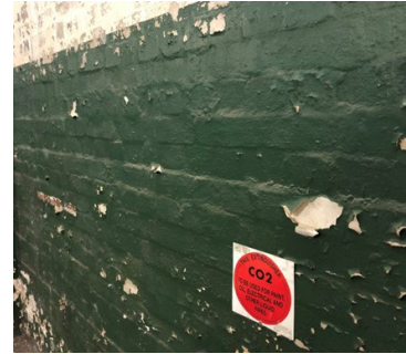
Lead paint on substation wall
