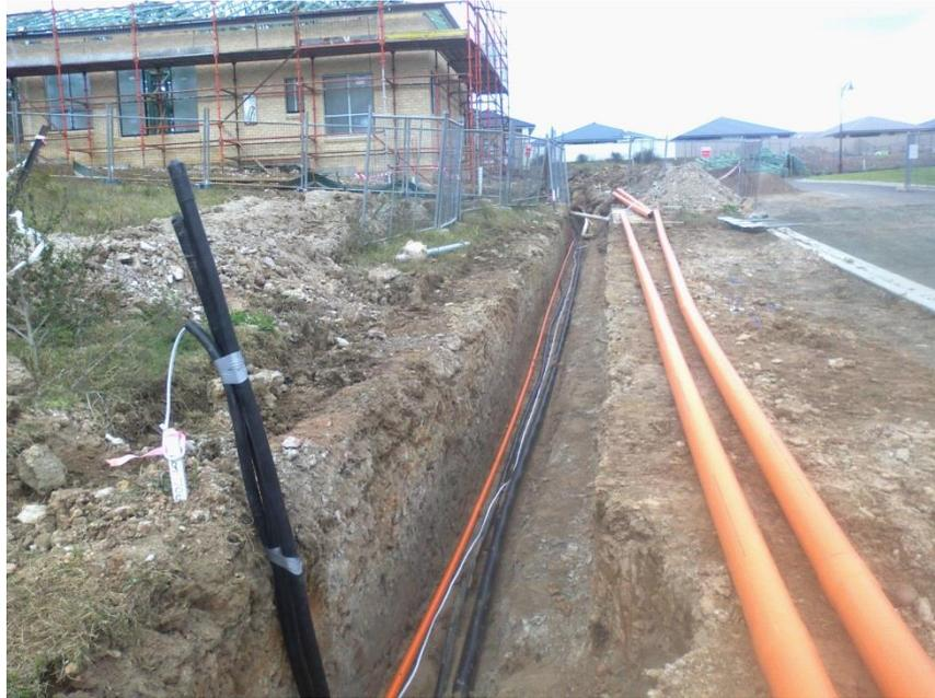
**Figure 32 LV cables turned up at boundary peg for future pillar**
