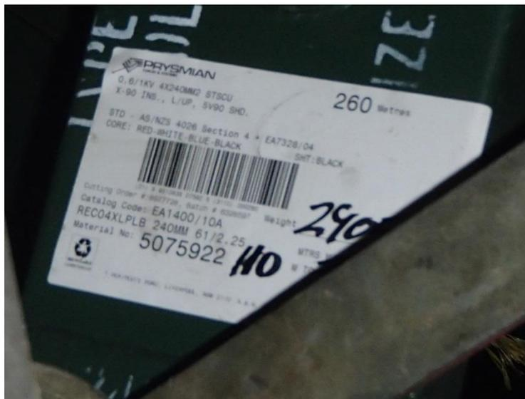
Figure 41 Cable drum details
