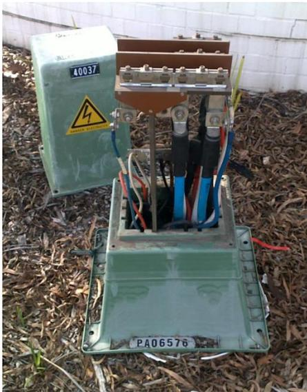
Figure 53 Double links – horizontally aligned
