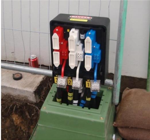
Figure 51 Double links - vertically aligned
