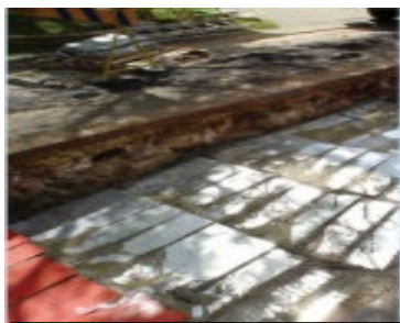
Cable trench with protective steel plates and orange PVC cover strip
