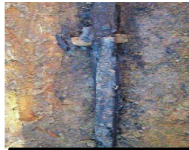
Direct buried bitumen encased cable chased into rock.
