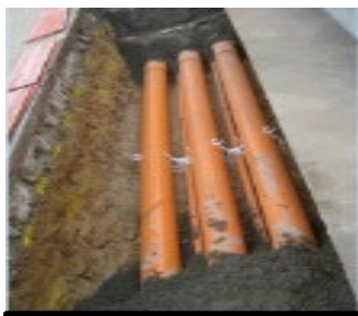
Open trench showing electrical conduits installed.
