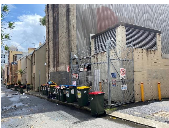
Figure 41. West facing view of Surry Hills Substation on Little Albion Street.
