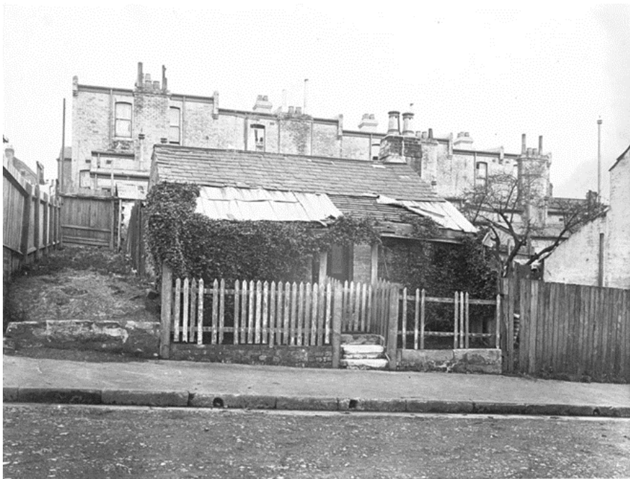
Figure 18. c.1910 photograph of 8 Smith Street, derelict Cottage, a brick and shingle-roofed cottage overgrown with ficus, with a battered wooden picket fence on raised sandstone and brick. Source: City of Sydney Archives.
