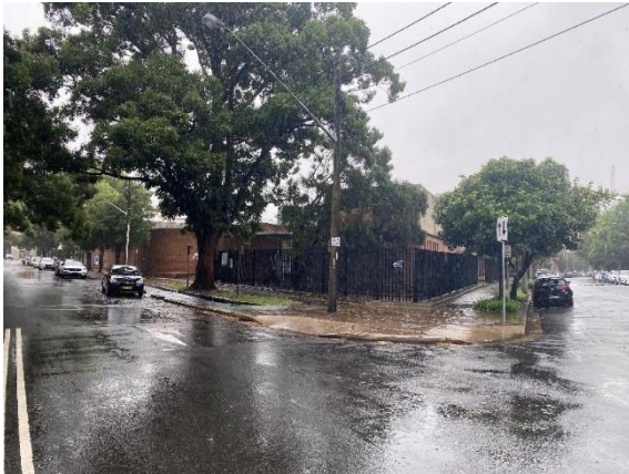
Figure 25. View to east of Zetland Substation and Allen Street.
