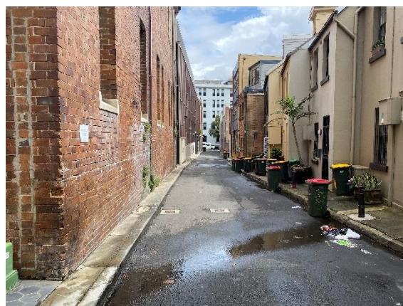
Figure 42. View to the west of Little Albion Street, including the rear of 80 Albion Street.
