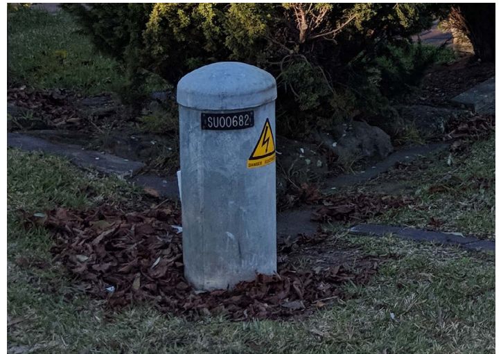
Typical pillar to be replaced
