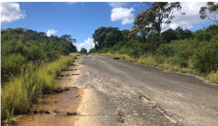
Ralston Avenue before works
