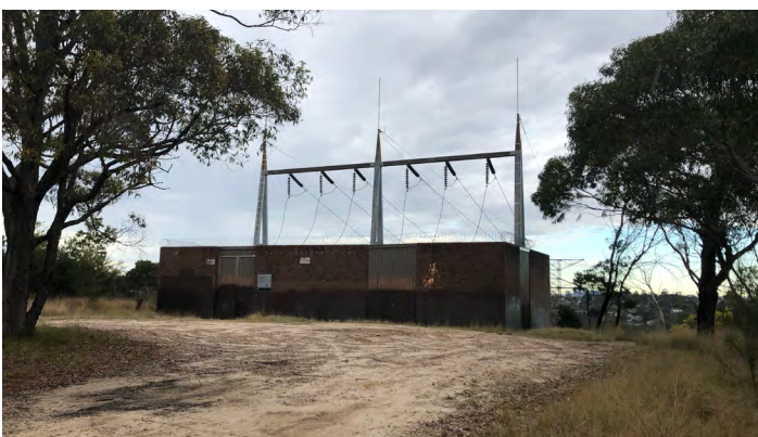
Western Lookout before works
