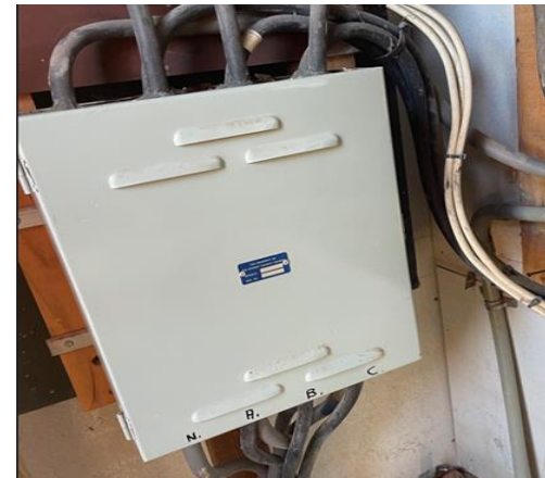
Image of metal clad service fuse cabinet
