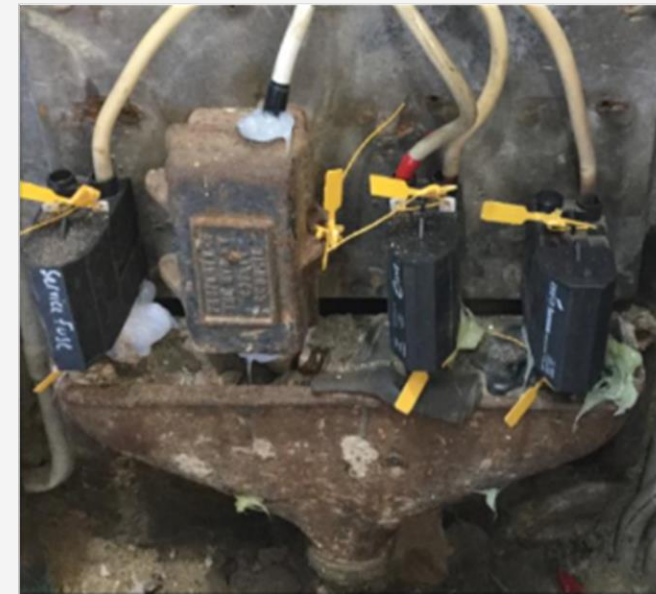
Images of metal clad service enclosures (handbag connections) with modifications completed
