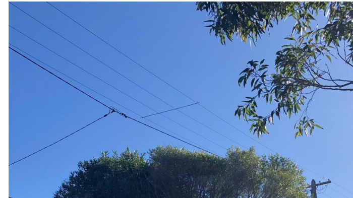
Images of 100Amp open wire mains suspended in span service
