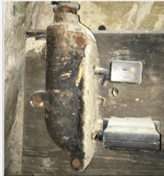
Images of metal clad service enclosures (handbag connections) with modifications completed
