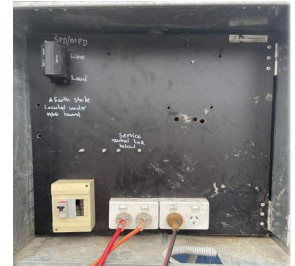
Image of Unmetered Supply
