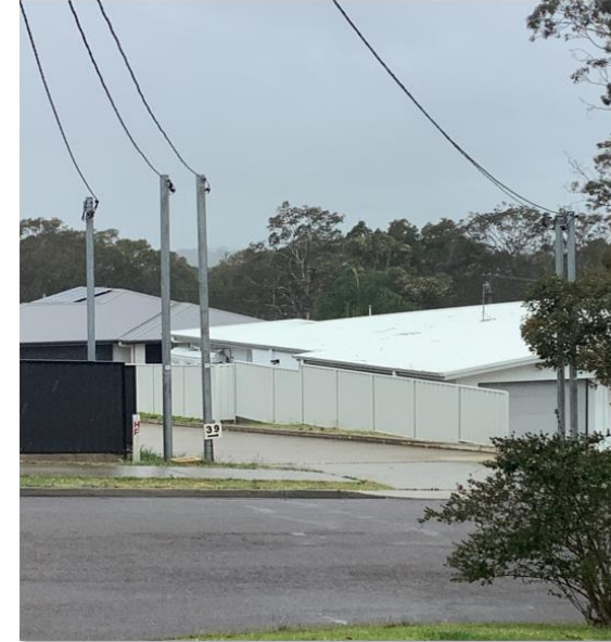
Image of Private poles installation on street
