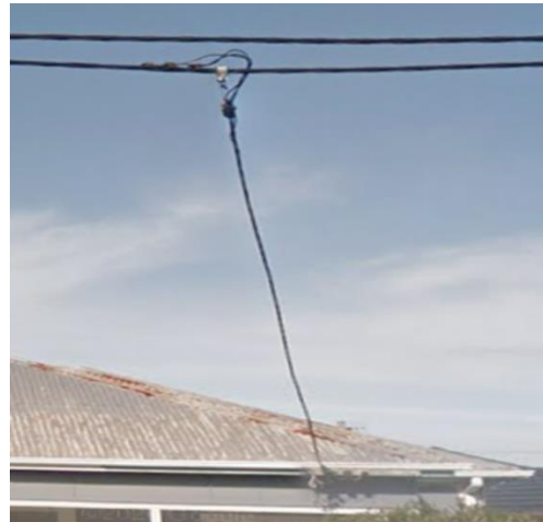
Images of Mid-span service from LVABC mains
