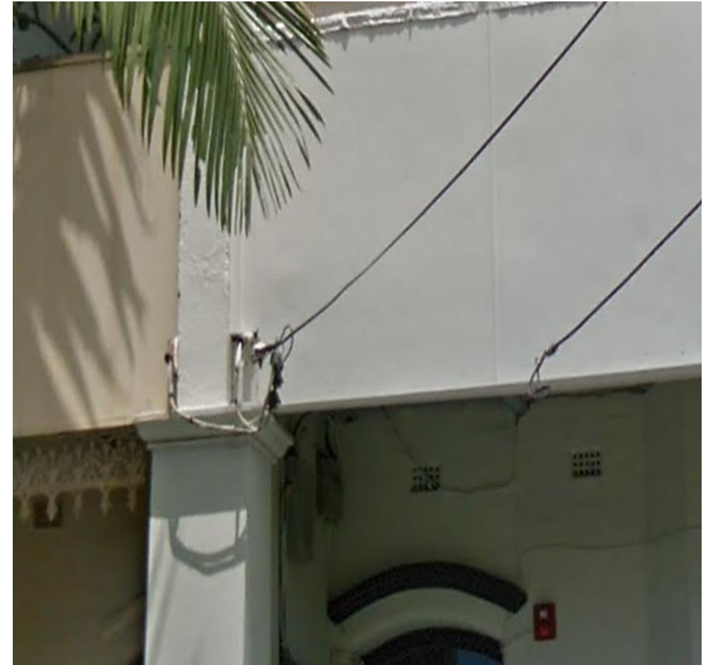
Image of Tap-off consumer mains connections
