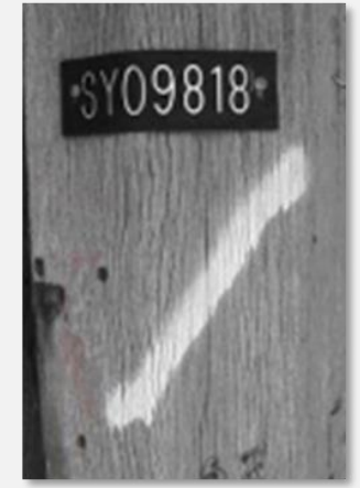
Image of Old defective pole marking
