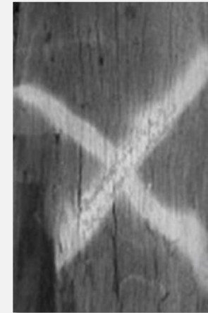
Image of Condemned pole cross
